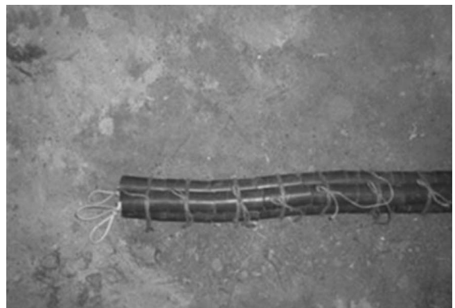
Fig. 9 Preparation of explosive before charging
